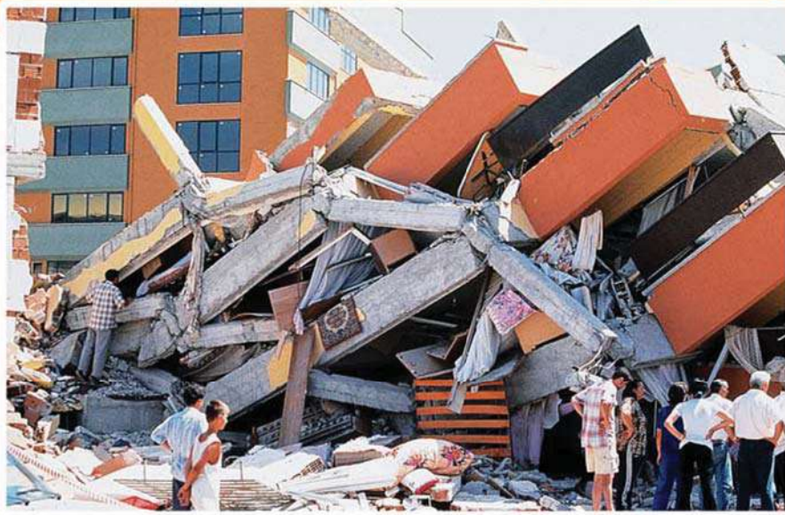
The quake destroyed 85,000 buildings. Many of the buildings were poorly constructed with inferior building materials. Floors of buildings “pancaked” and crushed the residents.
