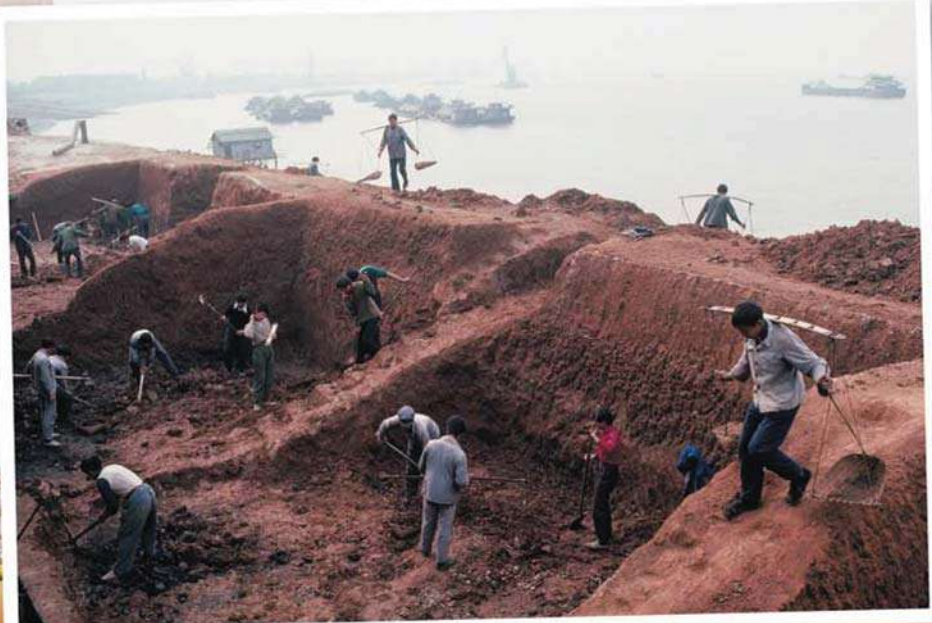
Along the Chang Jiang, human labor is still essential for flood control. These laborers work with shovels and other tools to fortify the banks of the river with dirt to prevent flooding.
