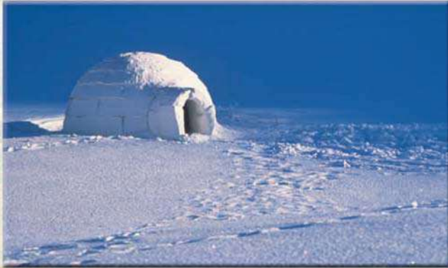
Arctic peoples in Canada and Greenland take advantage of their environment by using blocks of snow to build dome-shaped winter shelters called igloos. They sometimes add windows made with sheets of ice or seal intestines.
