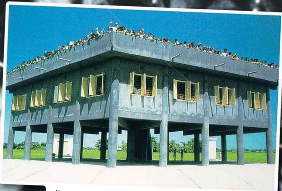
Concrete shelters constructed on stilts, as shown here, and reinforced school buildings are refuges from high floodwaters and winds that can knock down all but the strongest buildings.
